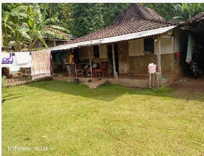
Figure 5: Sample of house conditions with low economic resilience in Balong Village: A semi-permanent house constructed entirely of wood
