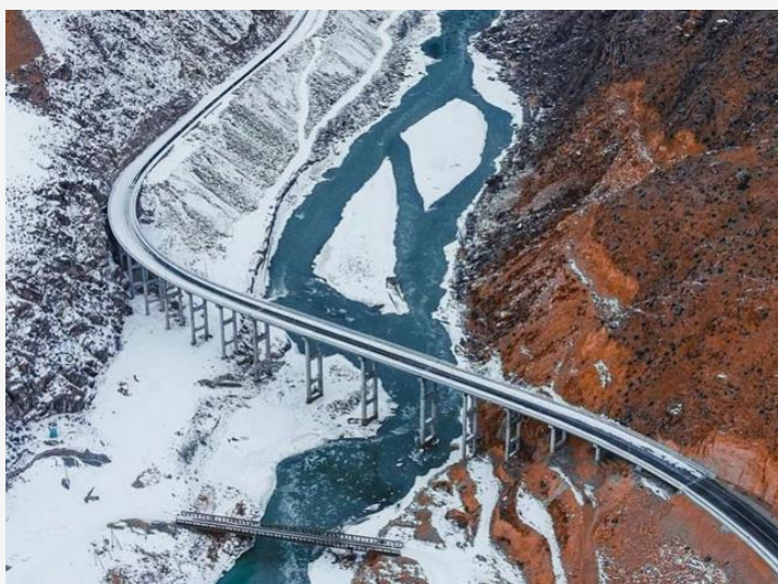
Figure 1: 396 m long bridge of the North-South alternative road
