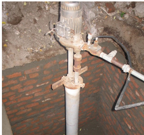
Figure 7: Bare pit for recharge purposes
