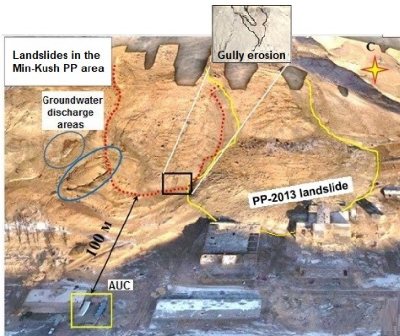
Figure 5: Landslide situation on the slope above the Min-Kush PP: UAV photography based 3D image of the slope and PP-2013 landslide (yellow outline); red dotted outline - the zone of active deformations of a new potentially dangerous landslide with a threat to the AUC; the gully areas are shown in the lower part of the dump in the black rectangle
