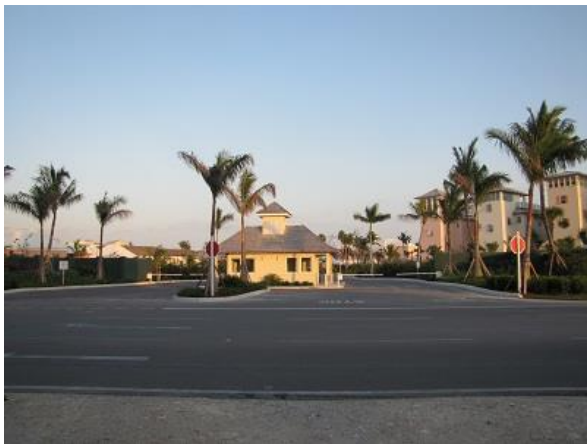
Figure 3: The gatehouse of Albany development.
