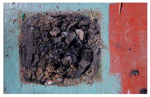
*It Almost Burned Down*—Consecutive images show burn area filled with cinders then cleared to reveal the damage through almost three inches of floor.
