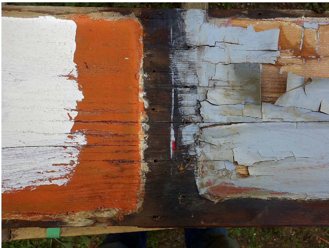
Ceiling —Removed twelve-inch-wide ceiling board shows various layers of paint.
