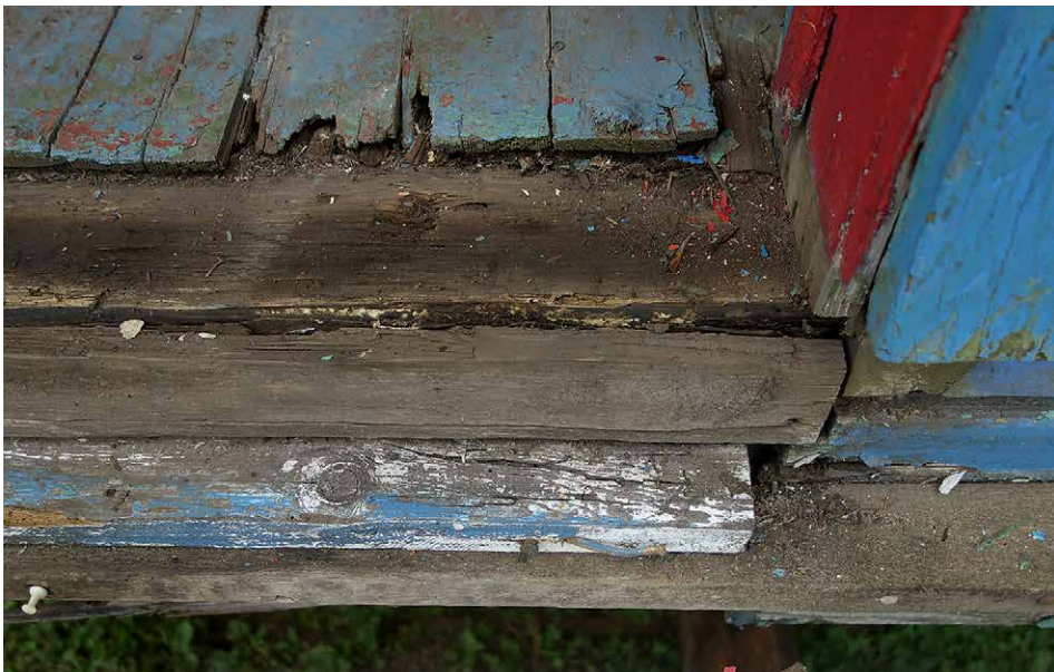
Threshold —Disintegration of the doorway evident after removing the sill.
